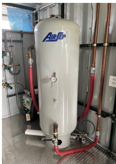
This oxygen receiver stores oxygen produced by the oxygen generator at Monapo District Hospital. Photo by Jan de Jong.
