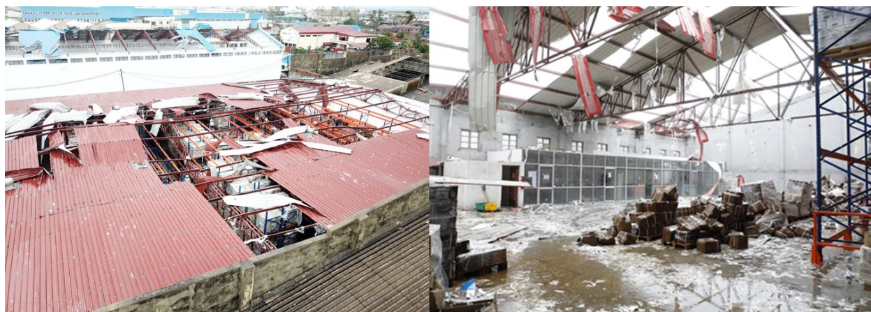
Warehouse Munhava in Beira, Mozambique, was one of the hardest-hit public health warehouses. The building needs major rehabilitation to be operational again, with a third of the roof missing and significant damage to one wall. Photo credit: Mickael Breard/GHSC-PSM
